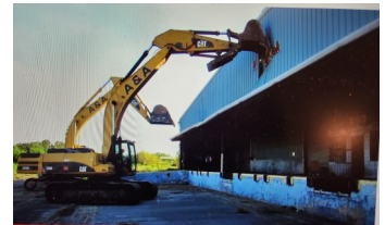
Ruth Reed drives demolition excavator *Source: Youtube
